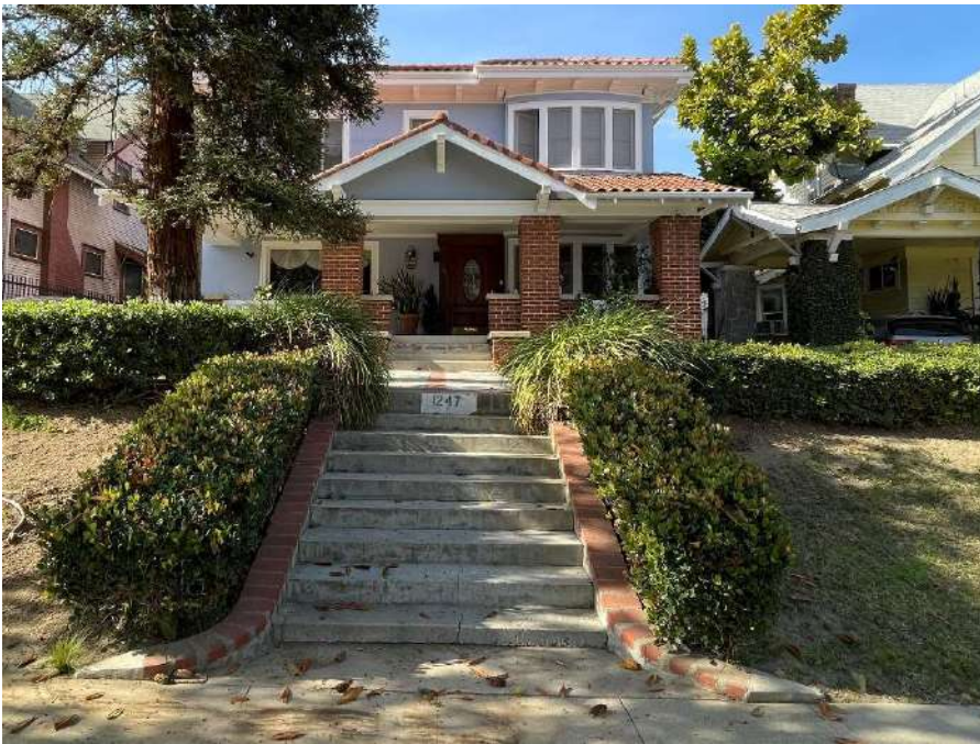
1247 S. Victoria Ave., facing west (typical contributor, built in 1926)
