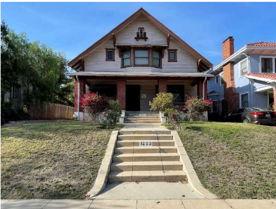
1253 S. Victoria Ave., facing west (typical contributor, built in 1908)
