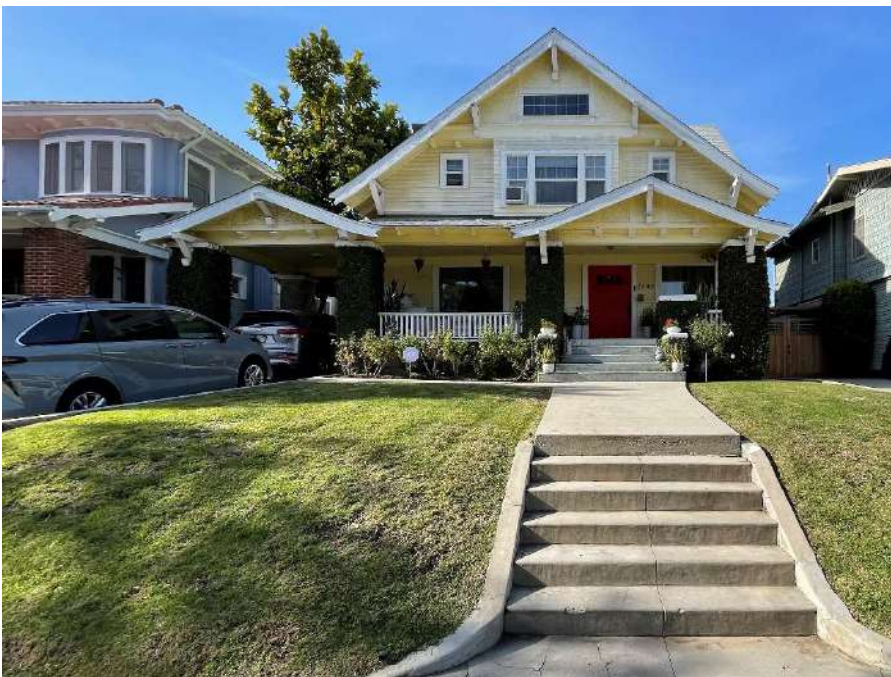
1243 S. Victoria Ave., facing west (typical contributor, built in 1909)
