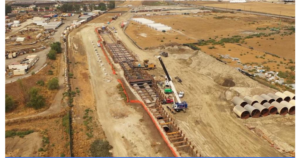
Installing earthquake-resistant pipes
