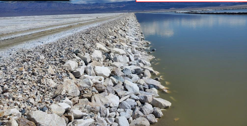
Protected 14.5 miles of berm slopes with Rip Rap
