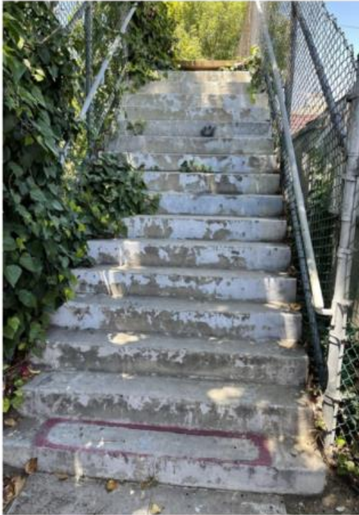
19. 000758 - Doman Ave Pedestrian Bridge
