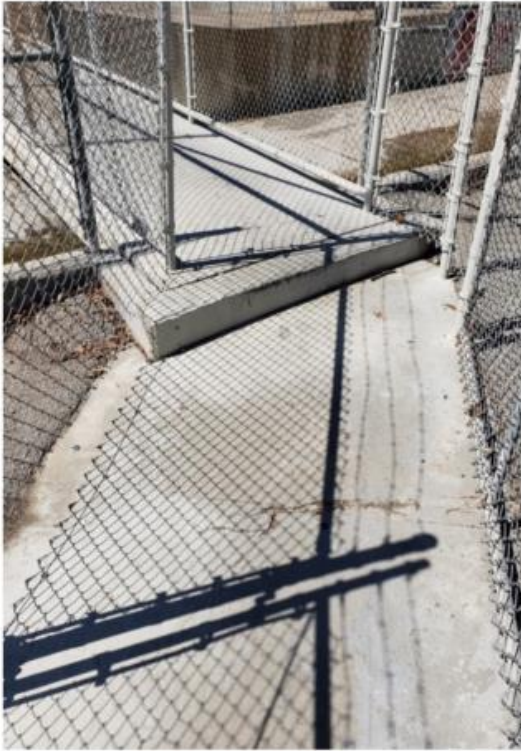
16. 000988 - Arminta St Pedestrian Bridge
