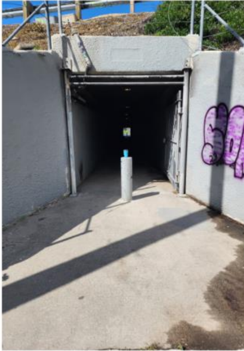
01. 531380 - Ediwanda Ave Pedestrian Tunnel
