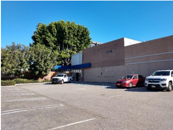
Photo #1 View of the site building (currently vacant) looking northeast.
