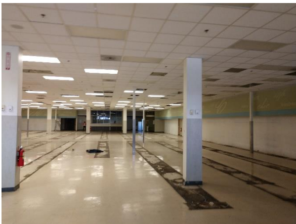
Photo #5 View of the interior of the site building which is current vacant.
