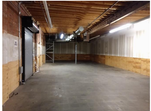
Photo #10 View of the southern portion of the site building.
