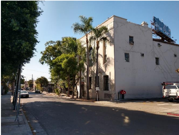
Photo #13 View of the southwest adjoining residential apartment complex.
