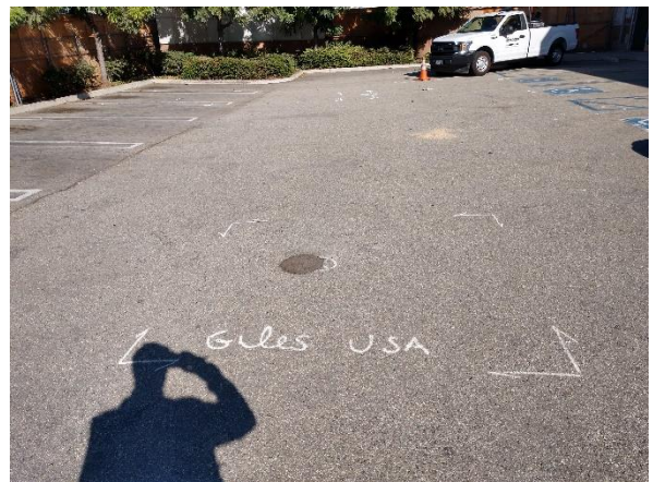
Photo #4 View of one of two exterior parking lot patches associated with previous site drilling activities.
