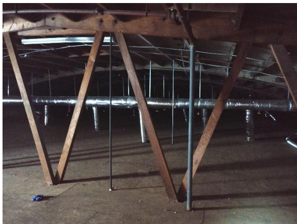
Photo #11 View of the second-story storage attic.
