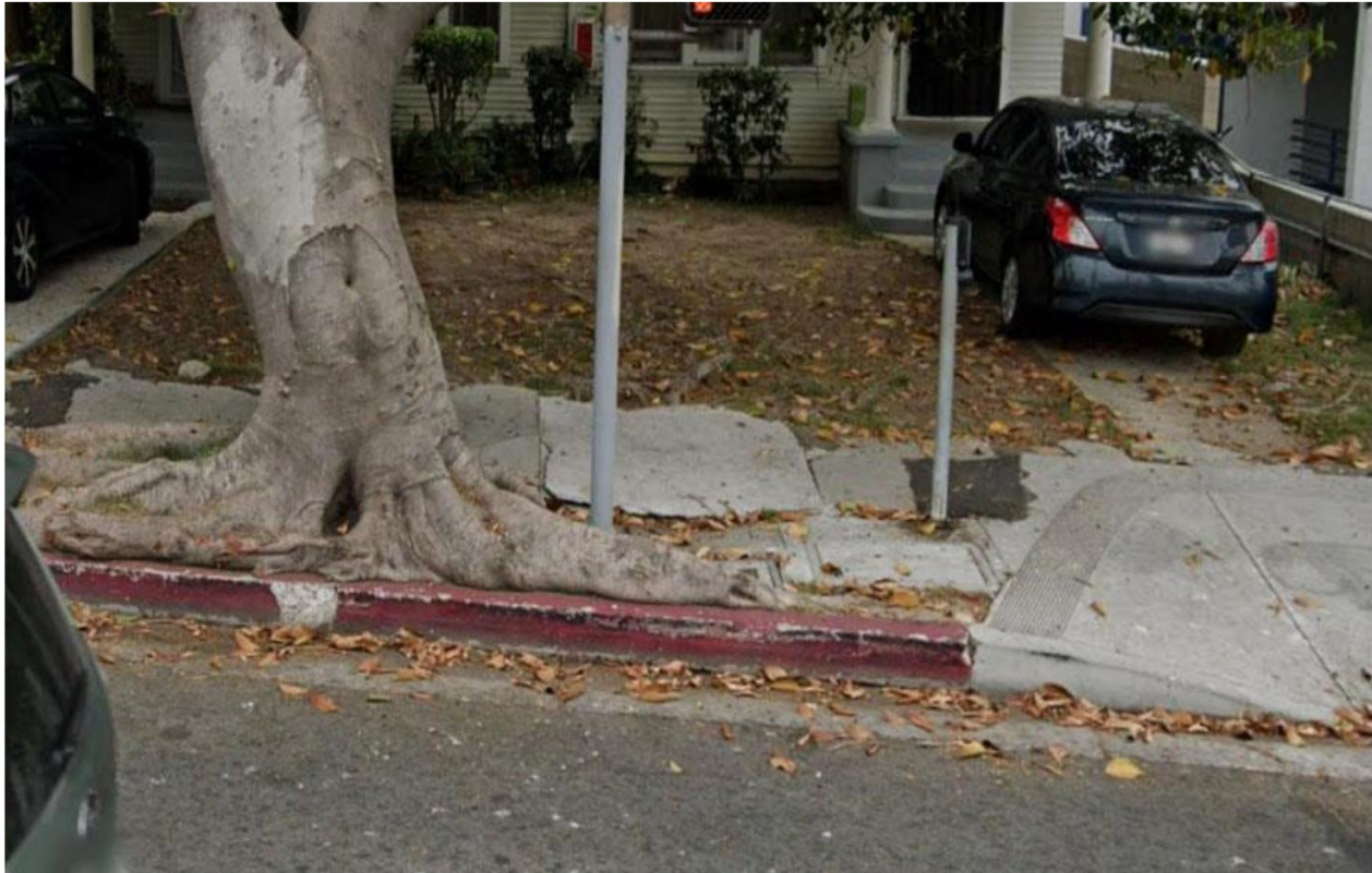
Figure No. 1: Existing Broken/Uneven Sidewalk at 5326 Fountain Avenue
