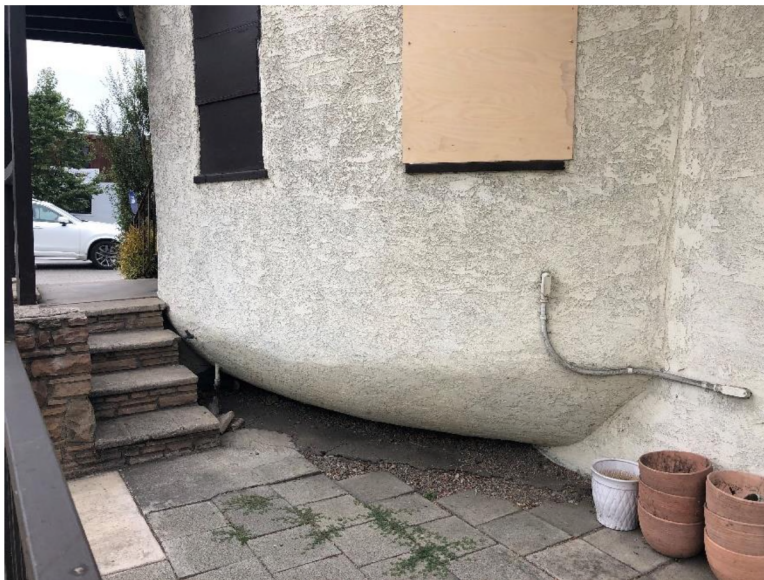
Figure 8. Detail of Rough Textured Stucco, Brick and Stone Veneer, and Boarded-Up Windows SOURCE: Sapphos Environmental, Inc., 2020
