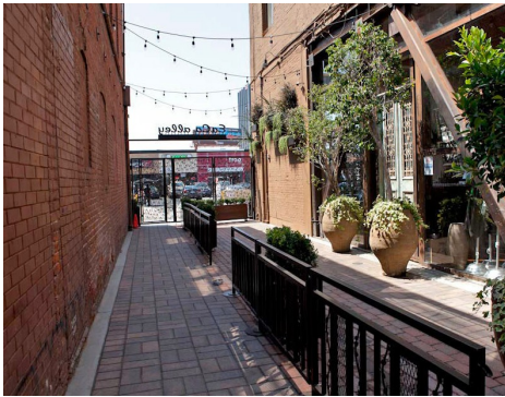
The East Cahuenga (“EaCa”) Alley is enhanced with permeable paving, outdoor seating, and nighttime lighting.
