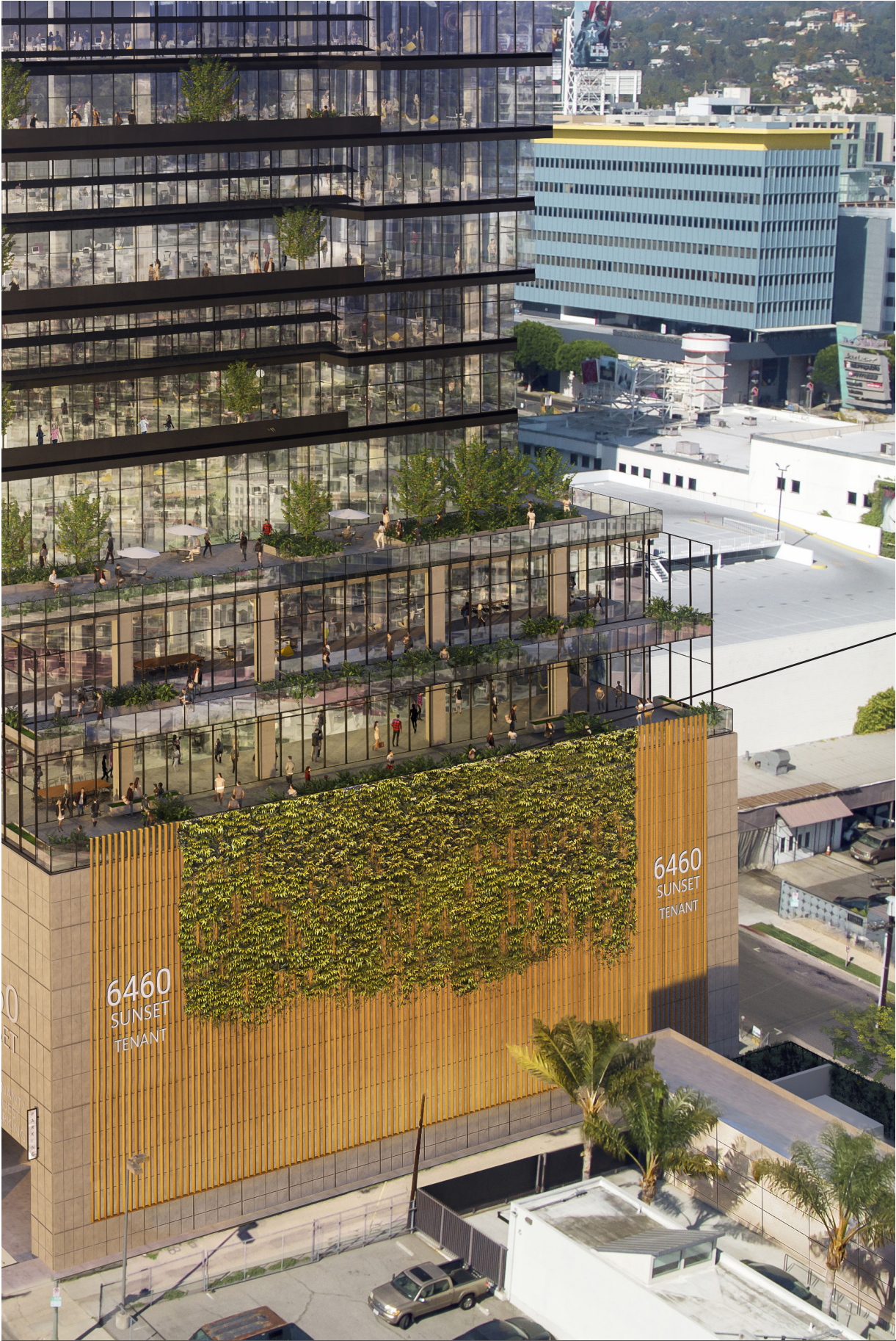
18" WIDE X 30" DEEP CONTINUOUS PLANTER, WITH INTEGRATED IRRIGATION
