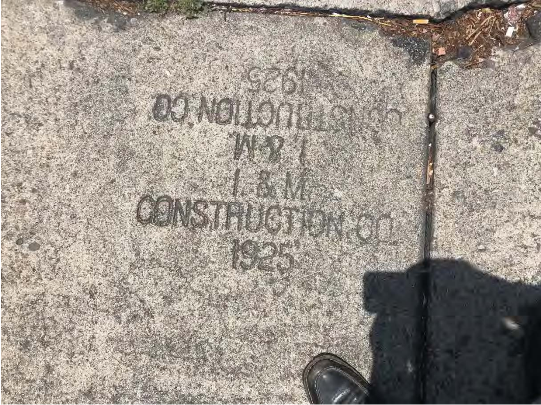
Concrete Slab in Carling Way Showing 1925 Construction Date
