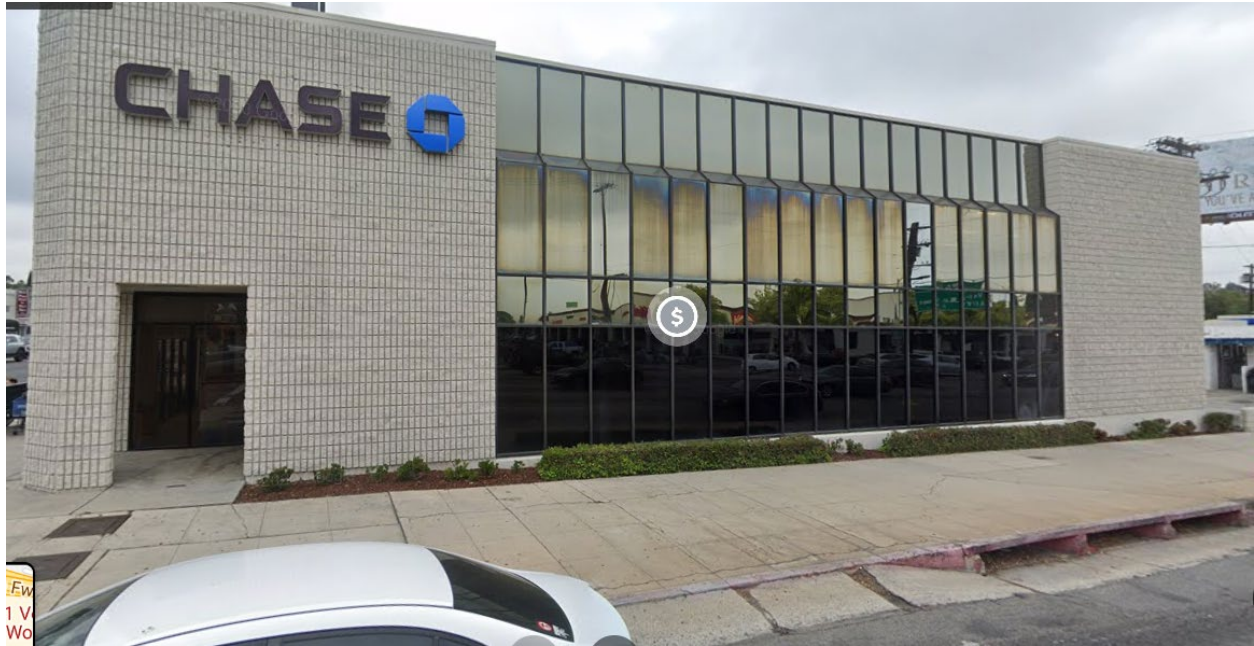
7. View looking at eastern frontage of subject site.
