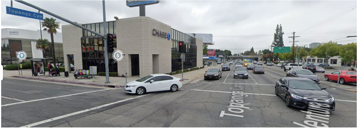
3. View looking northeast on Topanga Canyon Boulevard.
