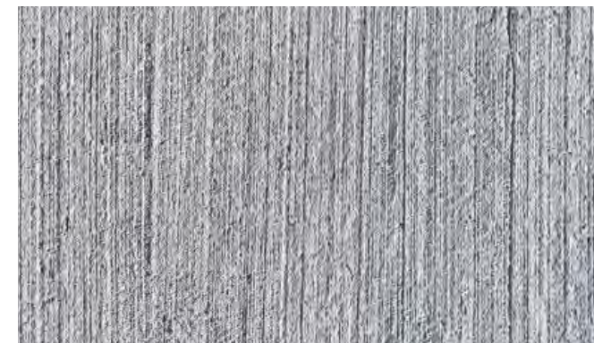
BROOM-FINISHED CONCRETE
