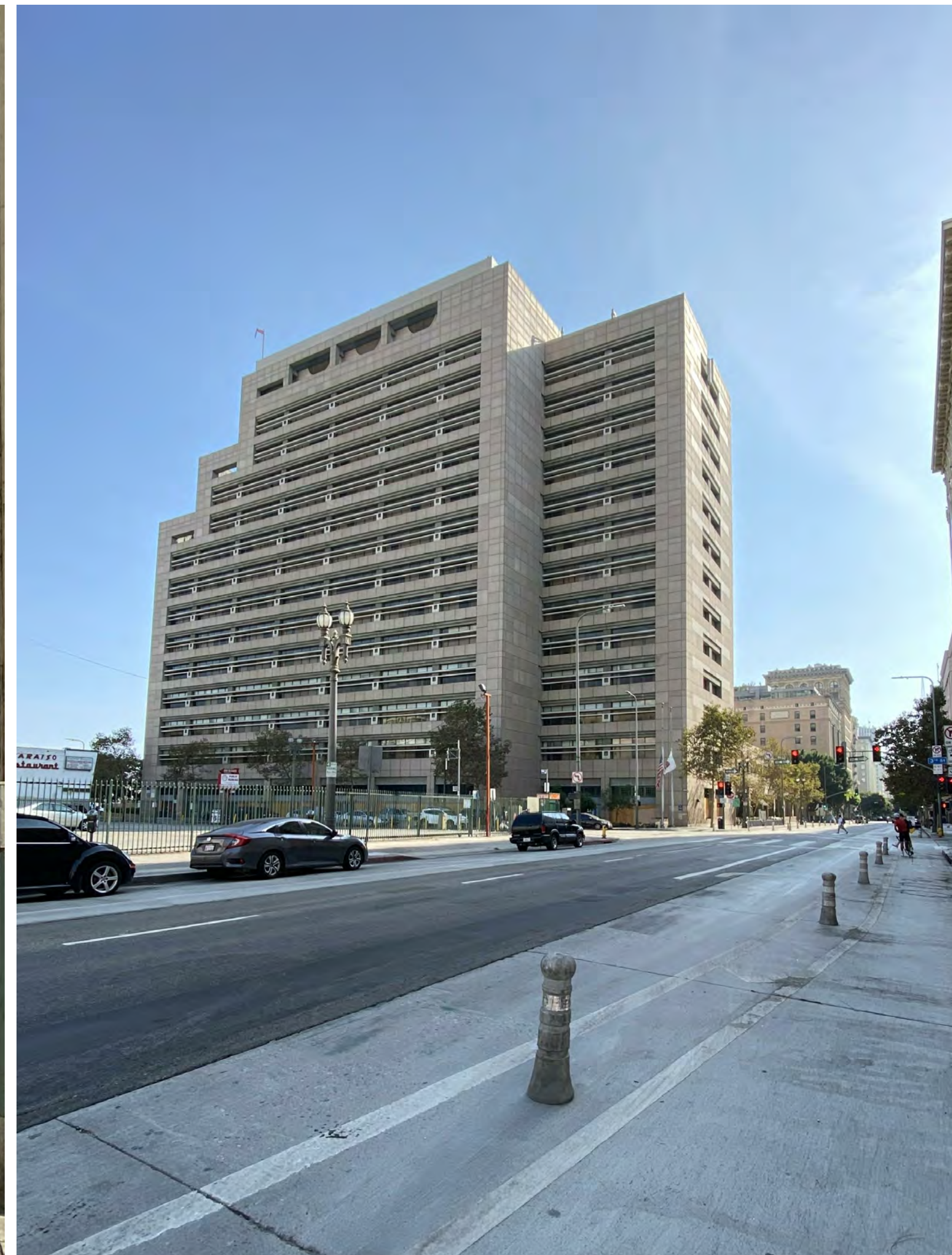
3. VIEW FROM NORTHWEST (SPRING STREET)
