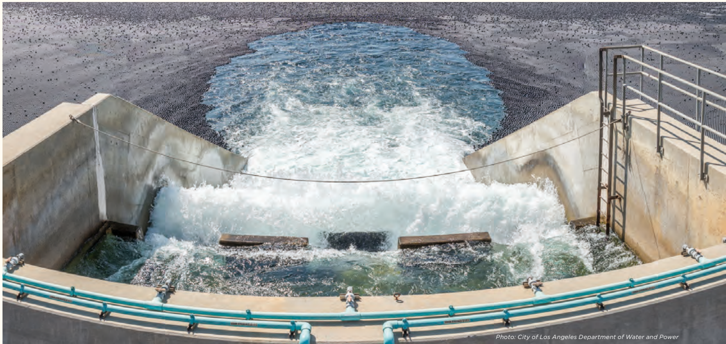
Photo: City of Los Angeles Department of Water and Power
