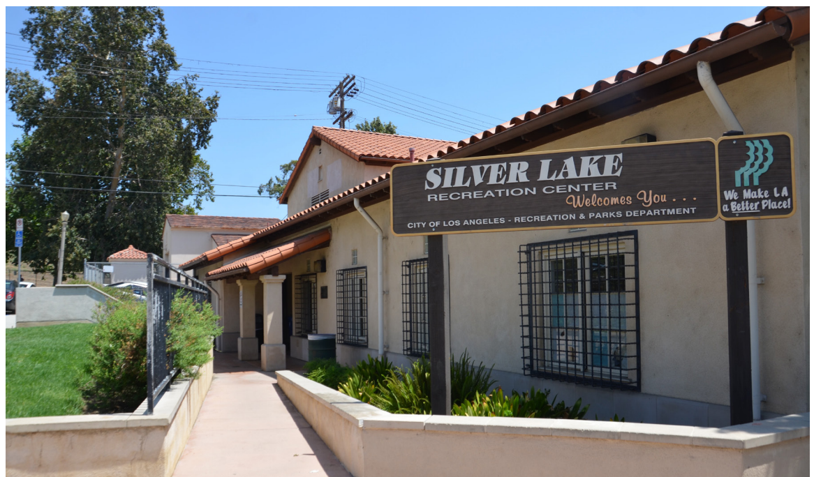
Figure 3-28 Existing Silver Lake Recreation Center entrance (right)
