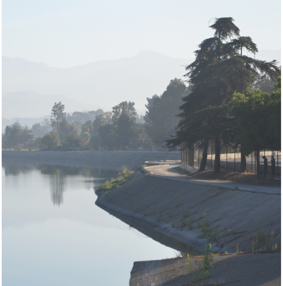
Figure 3-38 Inside the reservoir looking north along Silver Lake Blvd.
