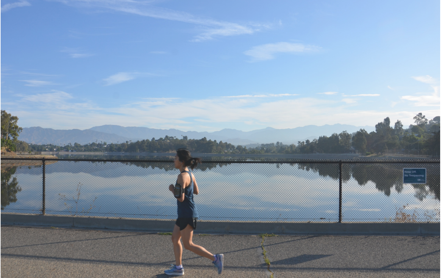
Figure 3-37 Runner along the South Dam Walkway
