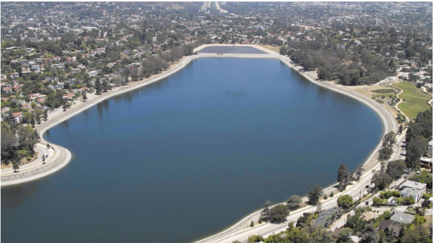
Figure 1-1 Image of The Silver Lake Reservoir Complex today
