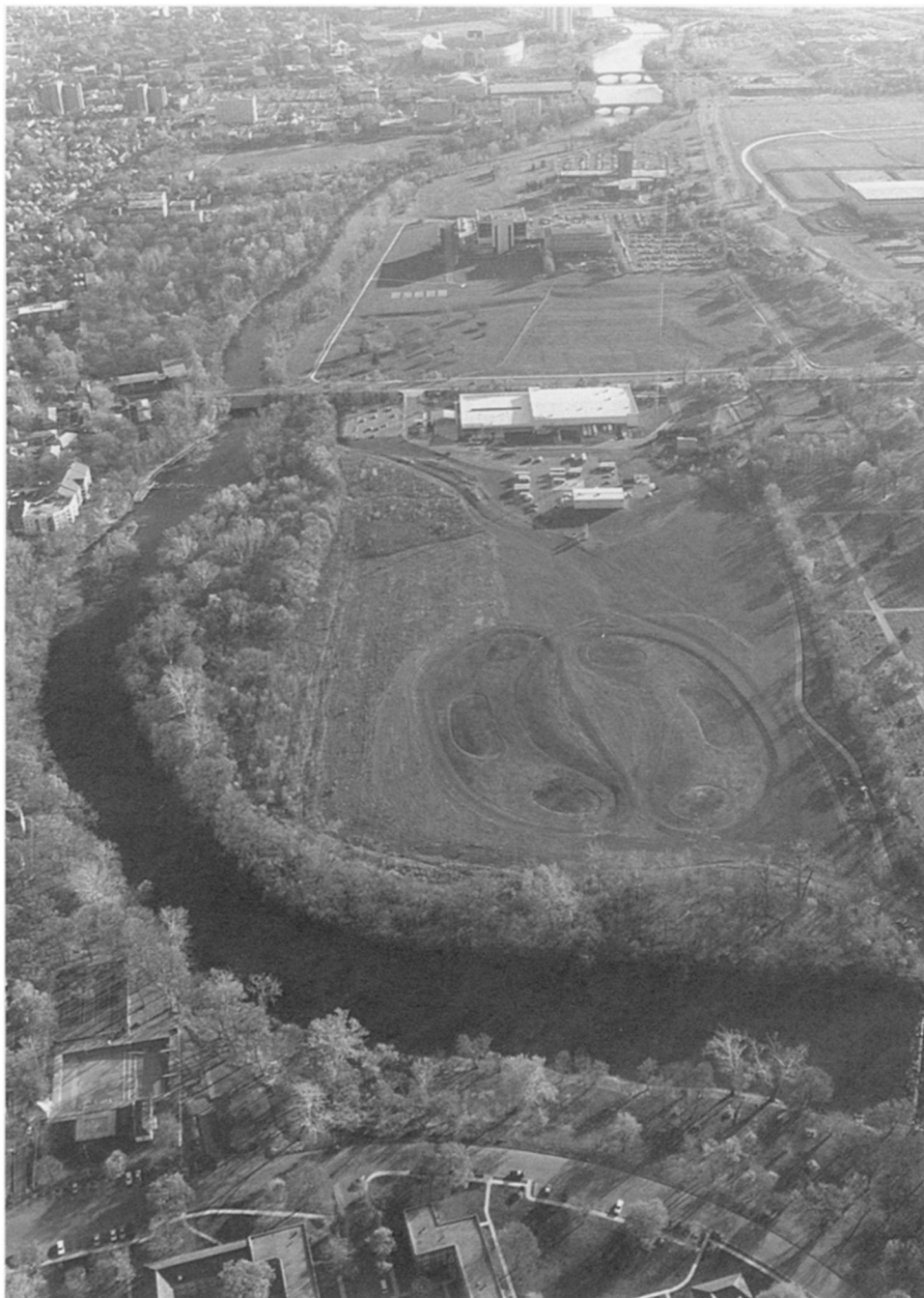
FIG. 3. The Olentangy River Wetland Research Park at The Ohio State University in Columbus, Ohio, USA, is a whole-ecosystem long-term experiment begun on 14 May 1994 with the planting of one of the deep-water marshes shown in foreground (right basin) with \approx 2500 plants representing 15 wetland species. The second deep-water marsh (left basin) remains unplanted. Each basin is 1 ha in size and water is supplied by pumps in the lower right-hand corner of the site to create a similar hydrology for each basin. The Olentangy River, shown flowing from bottom right to the top of the picture (with the university \approx 0.5 km downstream of the site on the horizon of the picture), is the source of the water, which is pumped in proportion to the river flow in the same patterns for each wetland basin. The photo was taken in November 1993 prior to the introduction of water to the wetlands (photo by Mark Myers, Apex, Columbus, Ohio).
