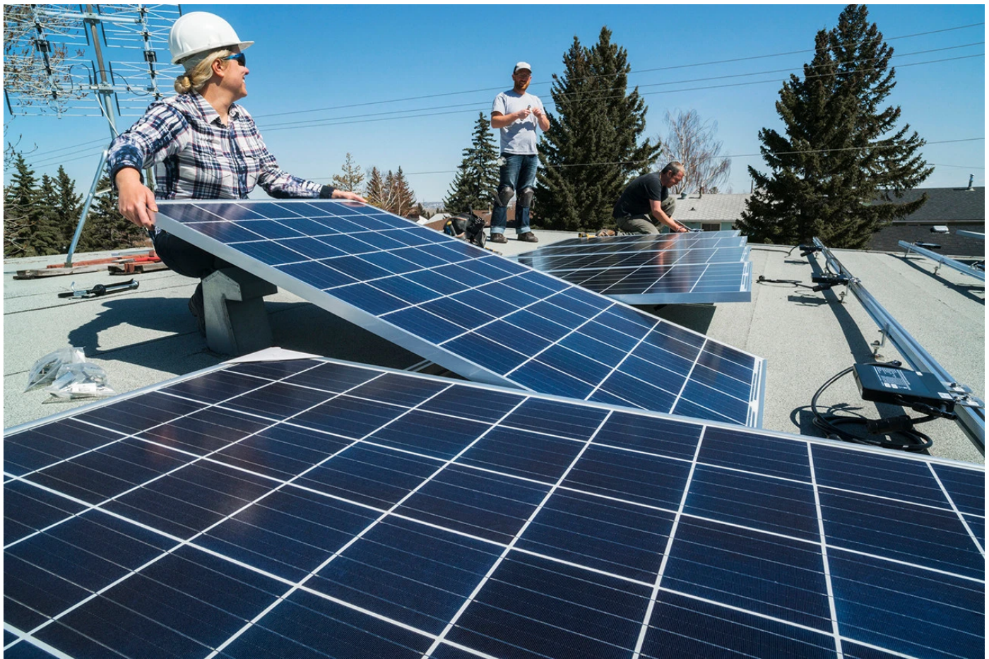
Workers installing solar panels on a residential homes roof.
