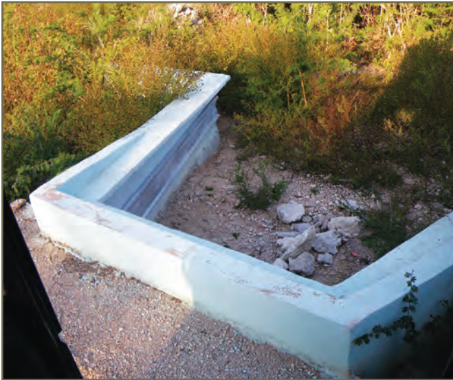
Photo 11. Tunnel with headwalls connected to concrete guide fencing in Cuba. © G. Barrett
