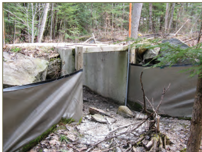
Photo 51. Fence tying into tunnel at Rice Lake Trail, Note shade cloth not recommended for permanent fencing © K. Gunson
