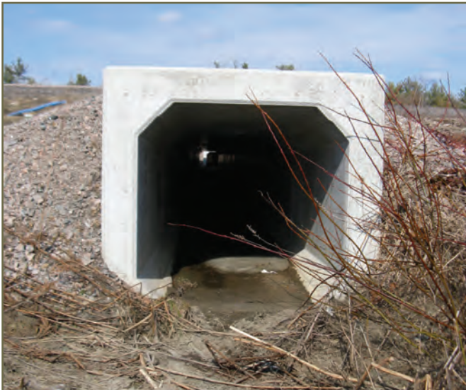
Photo 1. Precast box culvert along highway 69, Ontario. © K. Gunson
