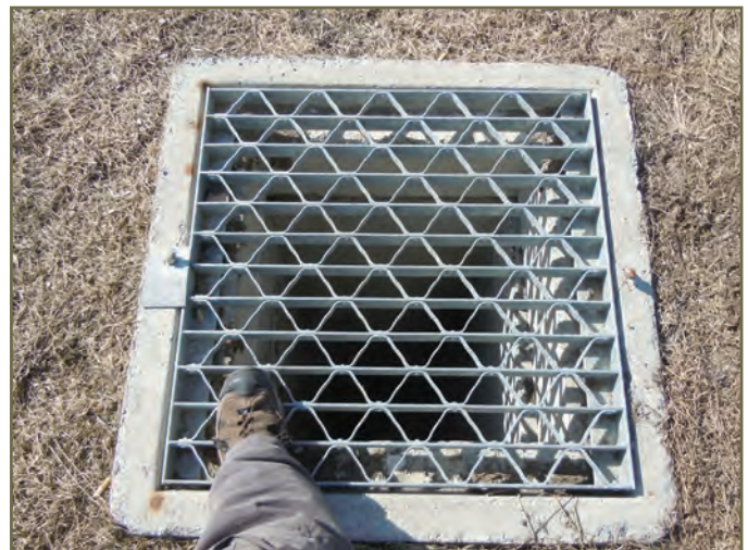
Photo 29. Zoom-in of skylight in median on Terry Fox Extension, Ottawa, Ontario. © D. Seburn
