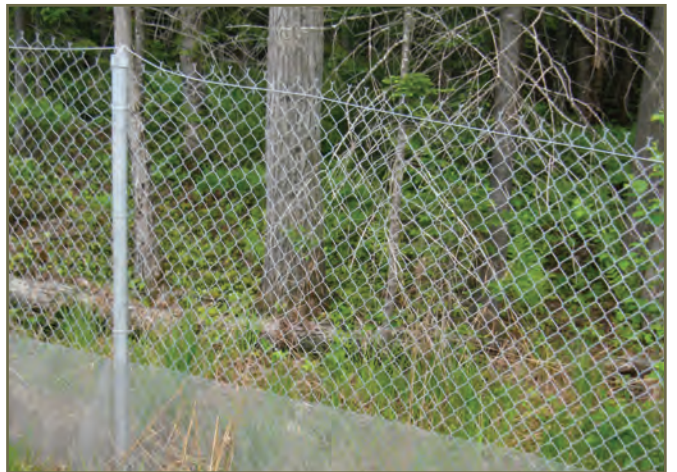
Photo 25. Small animal fence attached to the base of large animal barrier fence. © K. Gunson
