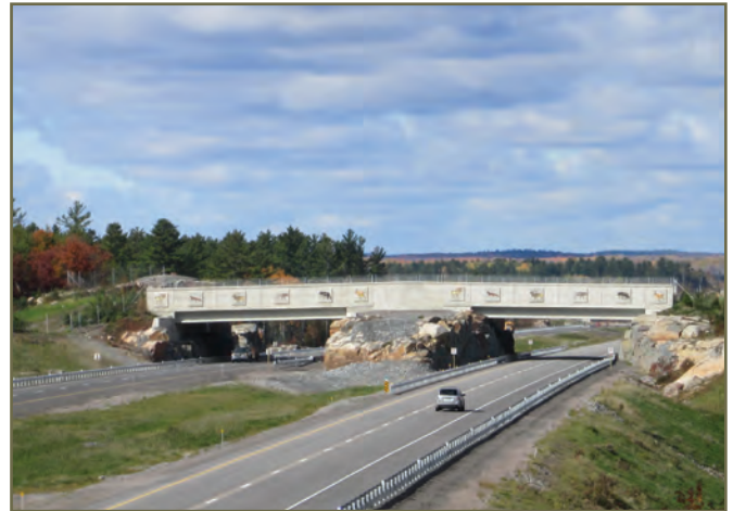
Photo 21. 30 m wide overpass installed near Sudbury on highway 69. © K. Gunson
