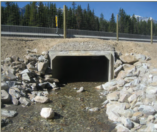
Photo 9. Open-bottom box tunnel with natural stream on Trans Canada Highway in Banff National Park, Alberta. © K. Gunson
