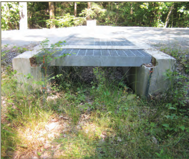
Photo 5. Open-bottom and open-top grate tunnel at Killbear Provincial Park, Ontario. © K. Gunson
