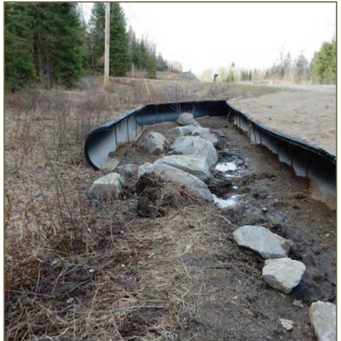
Photo 45. Fence end U design to deter animals following fence line from entering roadway in Haliburton County © K. Gunson
