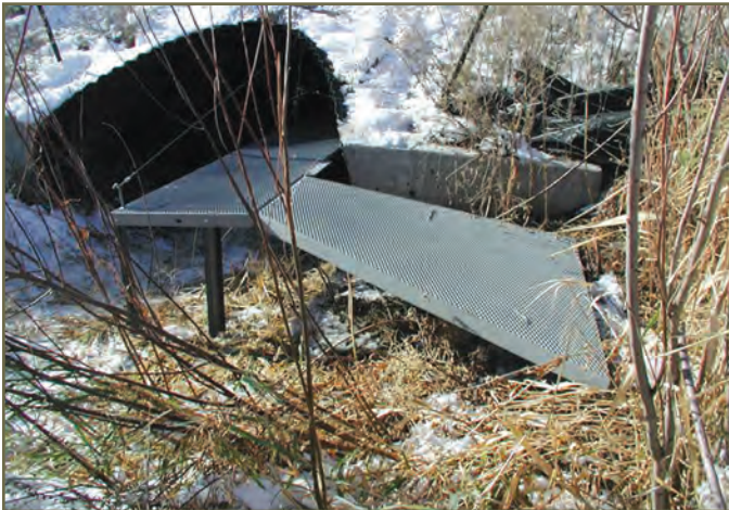
Photo 32. Dry bench in drainage culvert for small animals, could be modified for snakes. © K. Foresman
