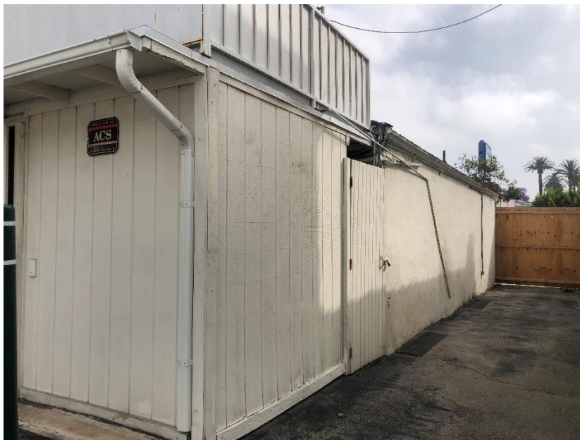
Figure 13. Southern Façade, 2113 Westwood Boulevard (view northeast) SOURCE: Sapphos Environmental, Inc., 2020
