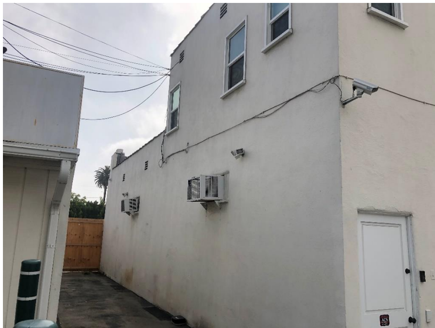
Figure 16. Northern Façade, 2115–17 Westwood Boulevard (view northeast) SOURCE: Sapphos Environmental, Inc., 2020
