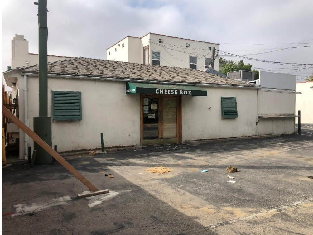
Figure 11. Northern Façade, 2113 Westwood Boulevard (view south) SOURCE: Sapphos Environmental, Inc., 2020
