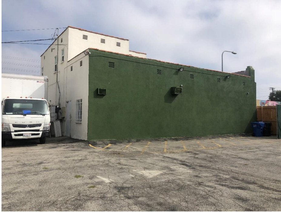
Figure 18. Southern Façade, 2115–17 Westwood Boulevard (view north) SOURCE: Sapphos Environmental, Inc., 2020
