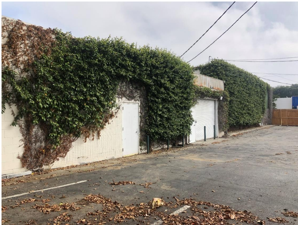
Figure 8B. Southern Façade, 2107-09 Westwood Boulevard (view northeast) SOURCE: Sapphos Environmental, Inc., 2020
