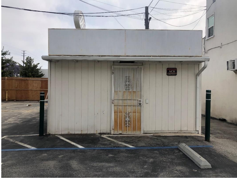
Figure 12. Southern Façade, 2113 Westwood Boulevard (view northeast) SOURCE: Sapphos Environmental, Inc., 2020
