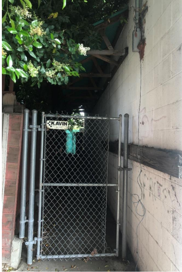
Figure 7. Western Façade, 2107–09 Westwood Boulevard (view northwest) SOURCE: Sapphos Environmental, Inc., 2020
