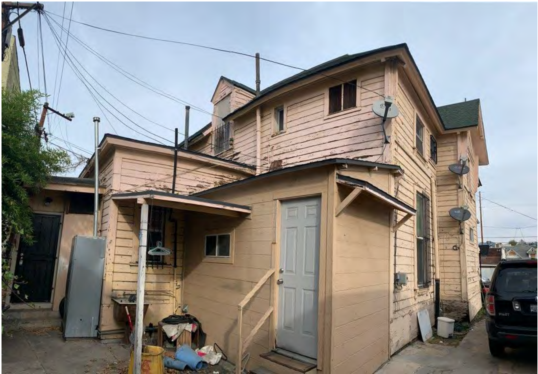
Rear (south) elevation, facing northwest. Photo by M. Rosalind Sagara.
