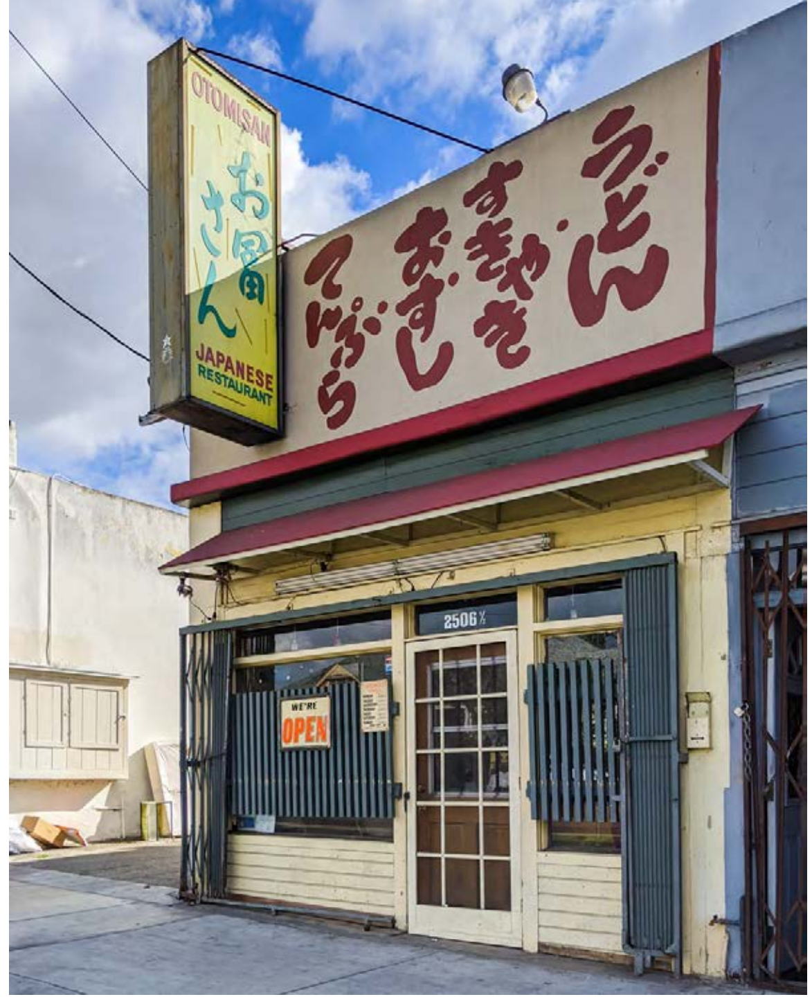
Primary entrance of Otomisan Japanese Restaurant, view facing southeast. Photo by Sue Hwang.
