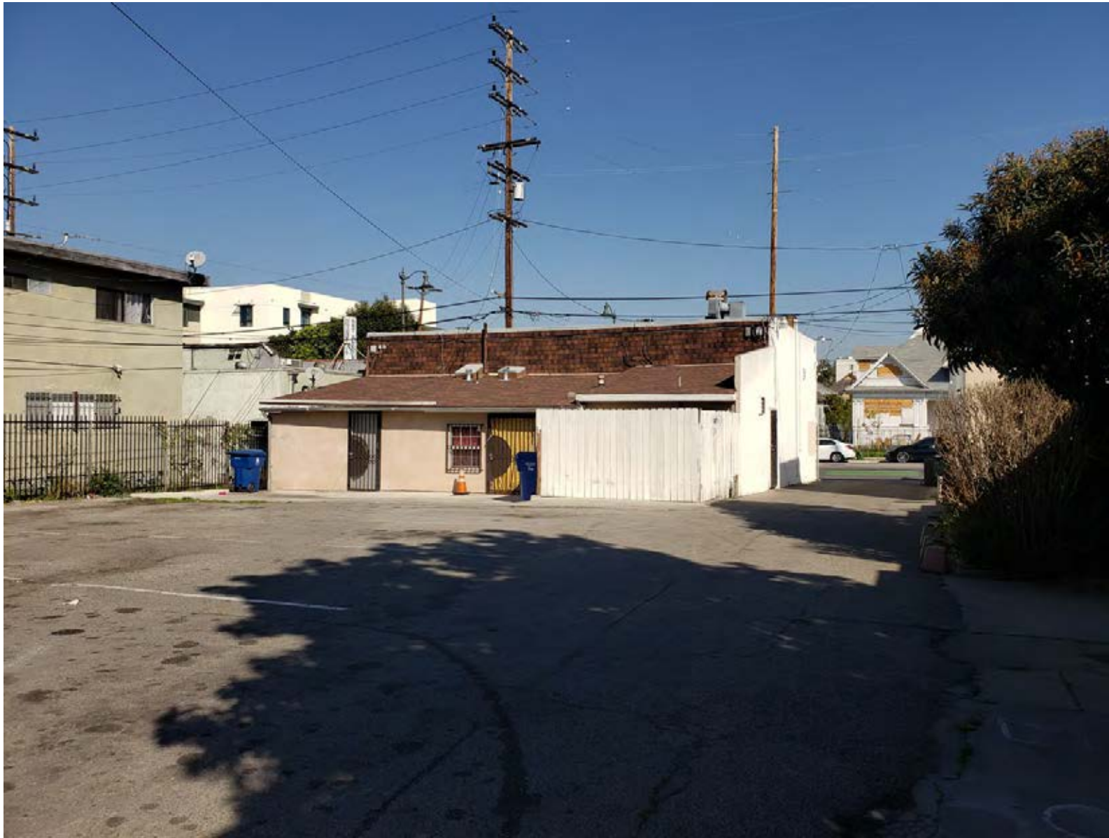
Rear (south) elevation of 2504-2506½ East First Street, facing northwest. Photo by M. Rosalind Sagara.
