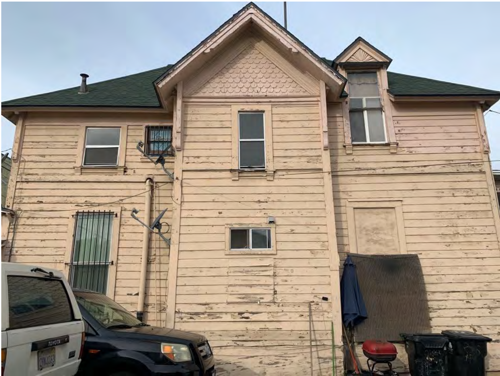
Secondary (east) elevation of 2508 East First Street, facing west.
