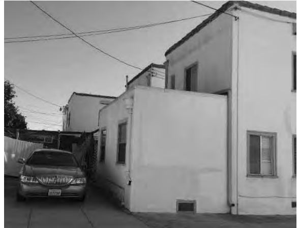
Figure 7: North elevation, looking east (GPA Consulting, 2019).
