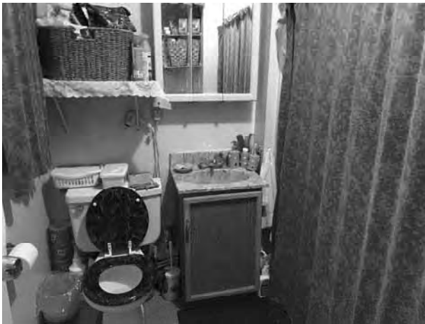
15. View of a typical restroom, in building A.
