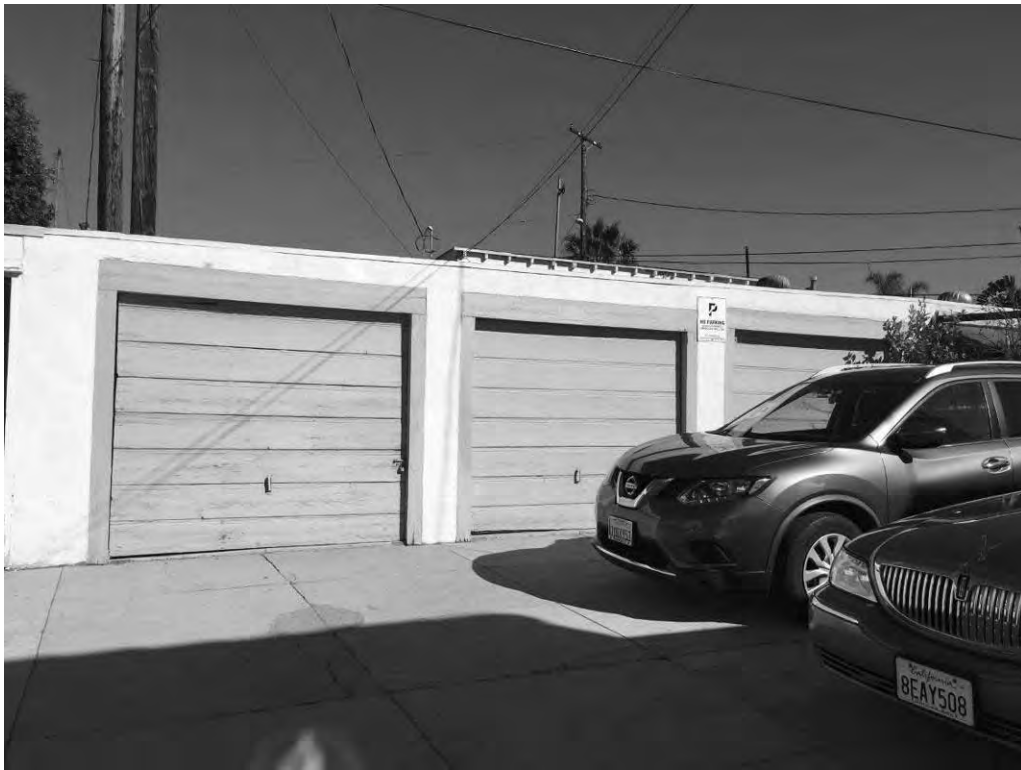
Figure 8: Detached garage, looking north (GPA Consulting, 2019).
