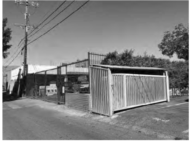
20. View transformer, on the north adjacent property.
