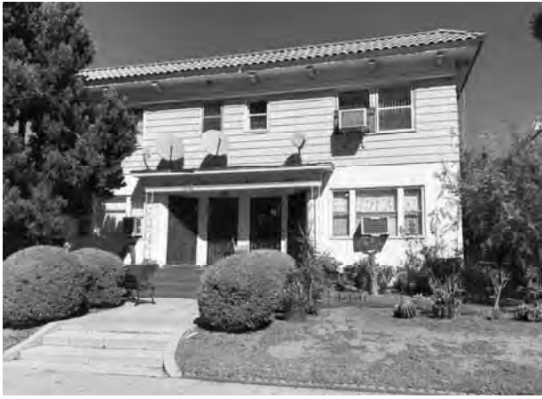
1. View of the south side of the subject property (building A), looking north.
