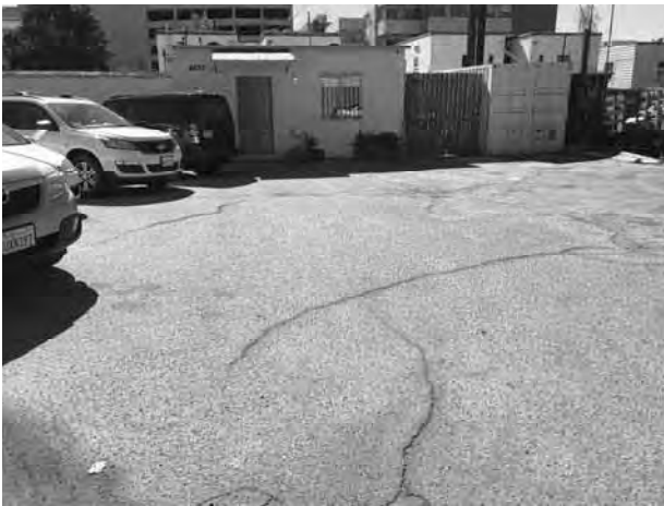
9. View of the north side of the subject property (building E), looking south.
