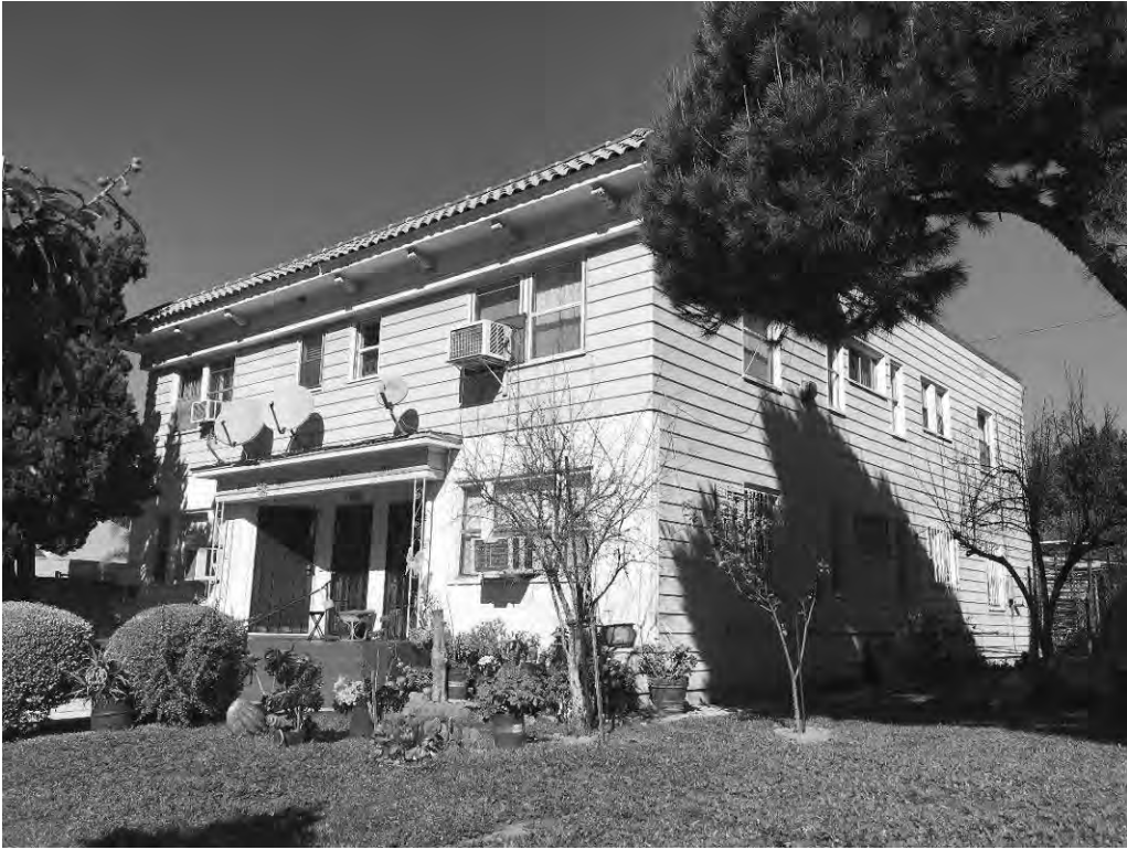
Figure 17: South and east elevations, looking northwest (GPA Consulting, 2019).
