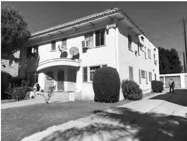
5. View of the south and east side of the subject property (building C), looking northwest.
