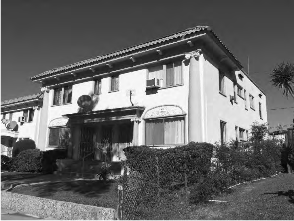
Figure 2: 4629-4635 Maubert Avenue, view looking northwest (GPA Consulting, 2019).
