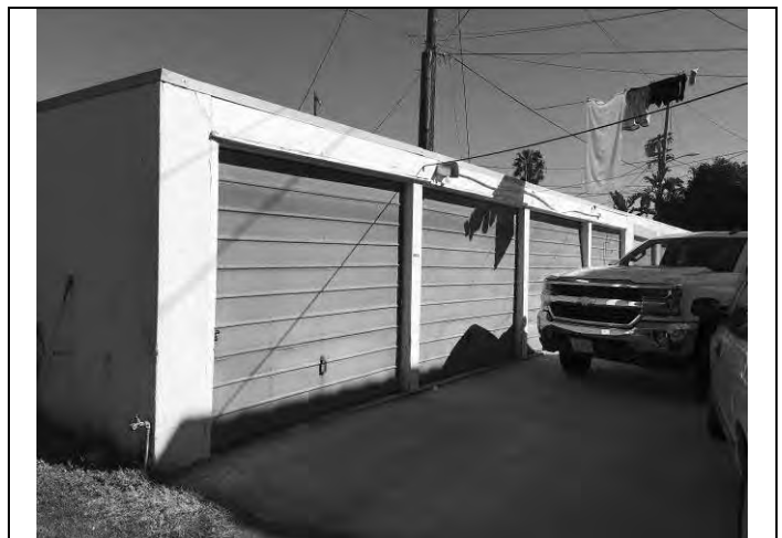
Image Detached garage, south elevation, looking northeast (GPA Consulting, 2019).
