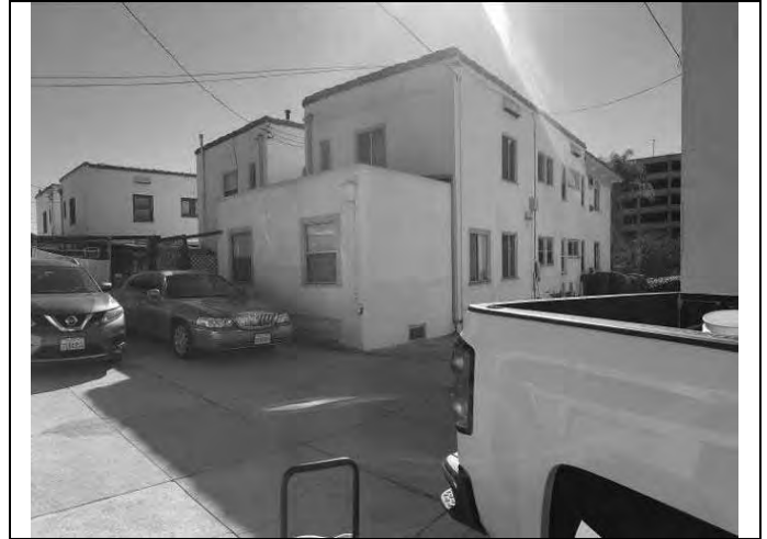
Image 4: North and west elevations, looking southeast (GPA Consulting, 2019).
