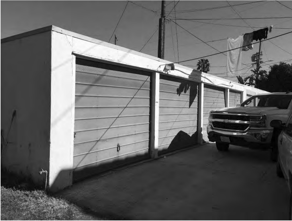
Figure 16: Detached garage, south elevation, looking northeast (GPA Consulting, 2019).
