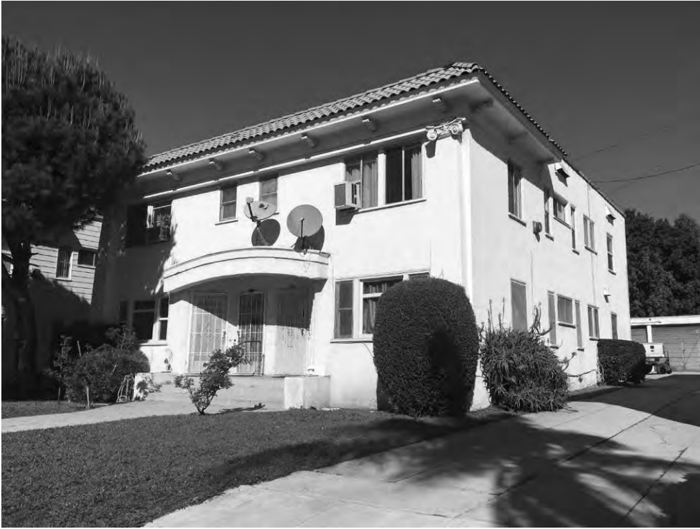
Figure 12: 4637-4643 Maubert Avenue, south and east elevations, looking northwest (GPA Consulting, 2019).
