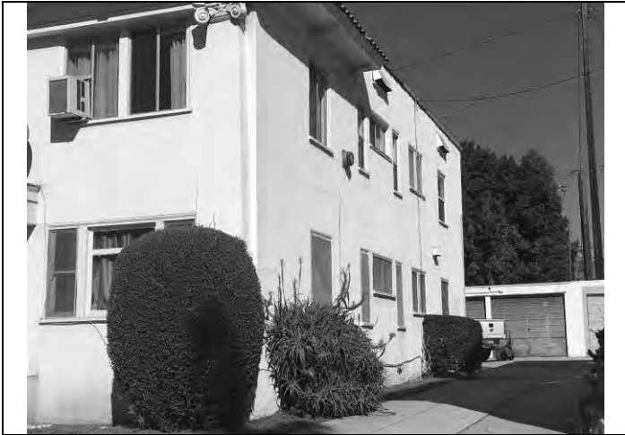
Image 1: East elevation, looking northwest (GPA Consulting, 2019).
