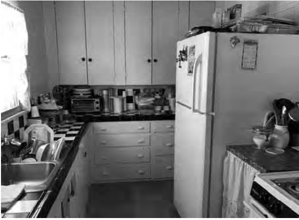
13. View of a typical kitchen, in building A.
