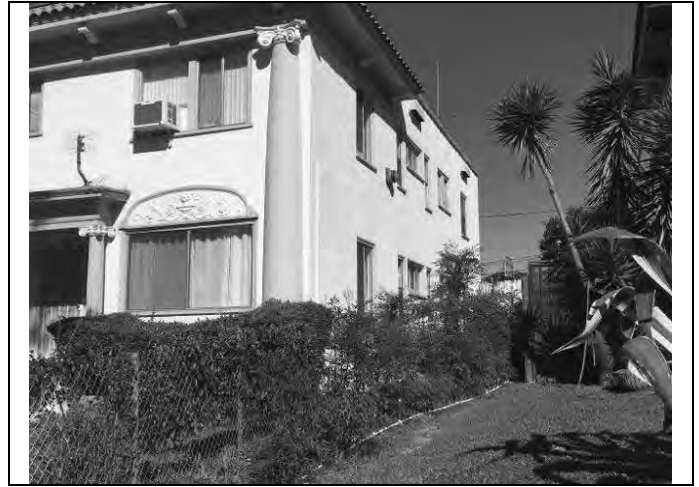
Image 2: East elevation, looking northwest (GPA Consulting, 2019).
