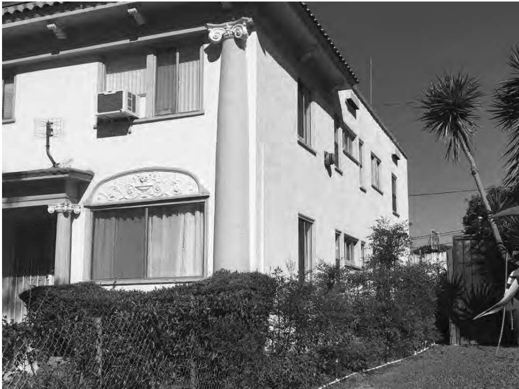
Figure 4: 4629-4635 Maubert Avenue, east elevation, looking northwest (GPA Consulting, 2019).
