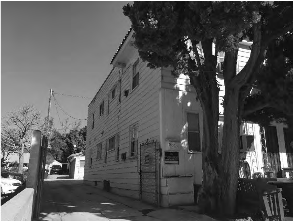
Figure 20: West elevation, looking northeast (GPA Consulting, 2019).
