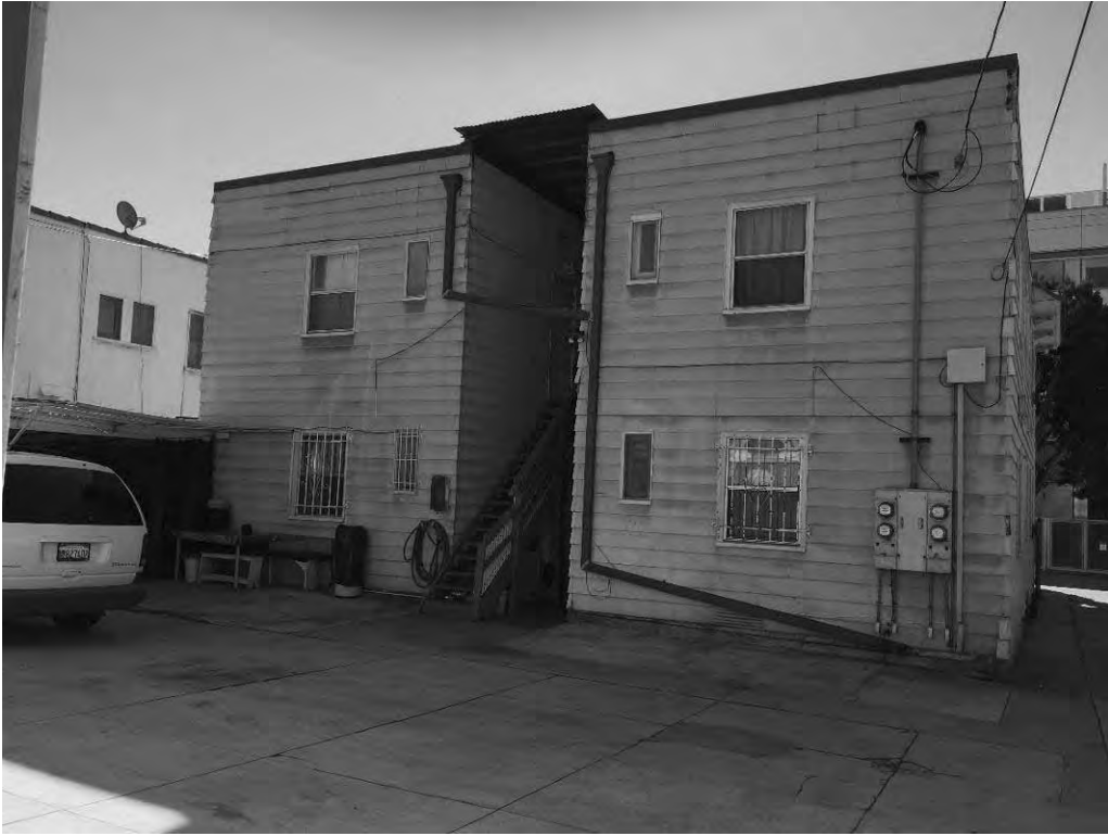
Figure 21: North elevation, looking southeast (GPA Consulting, 2019).
