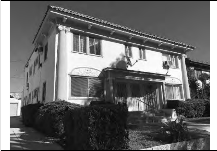
Image 1: South elevation, looking northeast (GPA Consulting, 2019).
