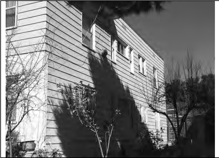
Image 1: East elevation, looking northwest (GPA Consulting, 2019)
