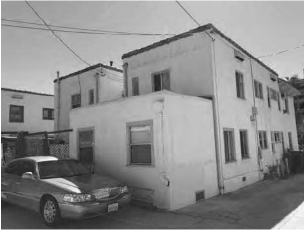
7. View of the north and west side of the subject property (building D), looking southeast.
