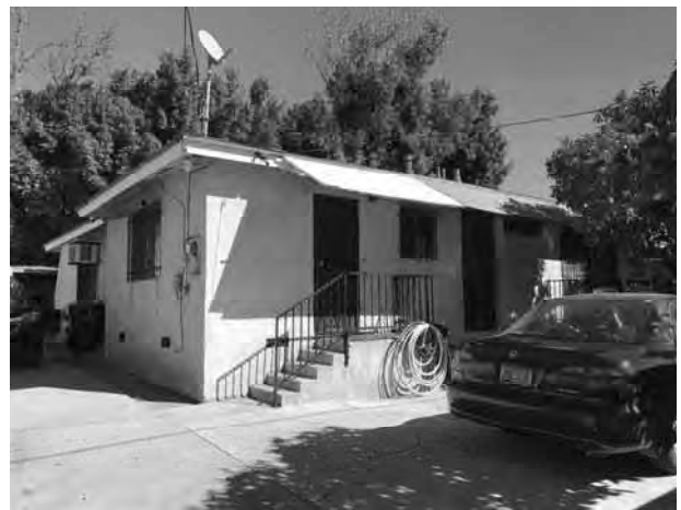
4. View of the south and west side of the subject property (building B), looking northeast.
