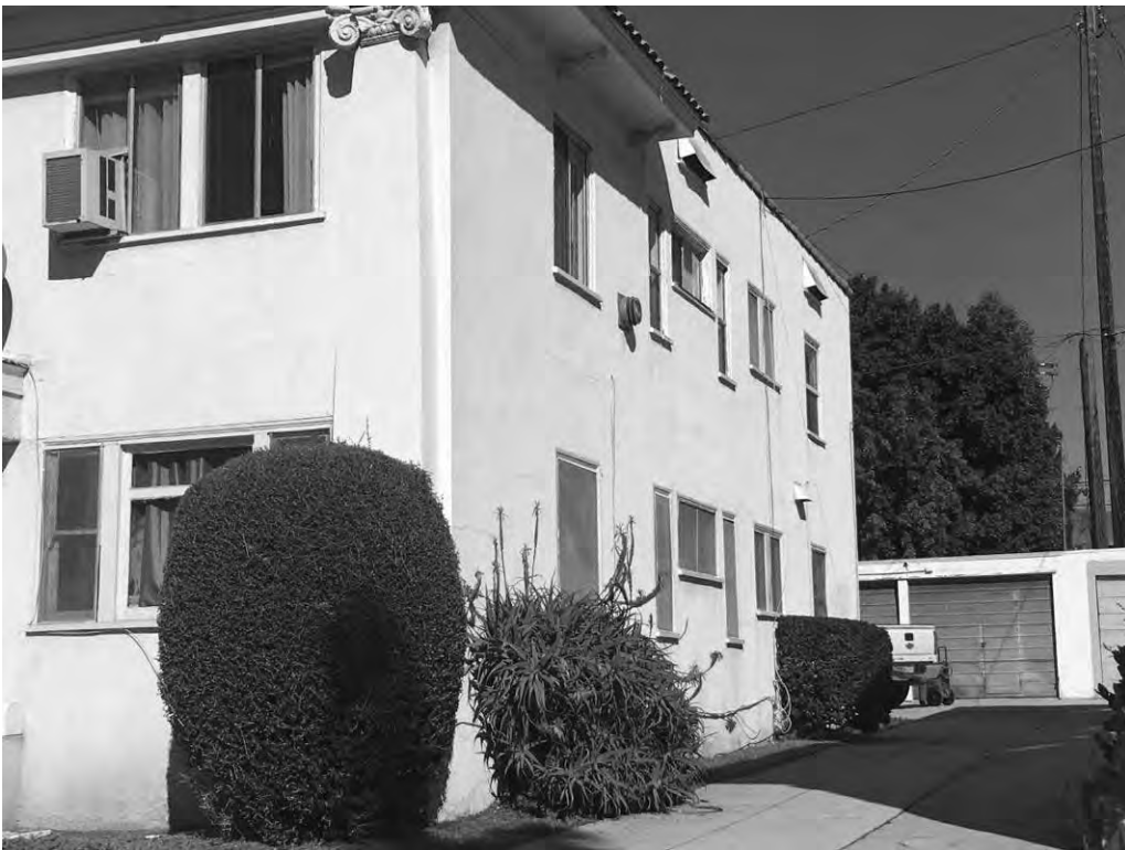
Figure 13: 4637-4643 Maubert Avenue, east elevation, looking northwest (GPA Consulting, 2019).
