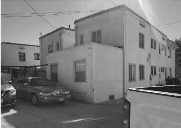
Figure 6: North and west elevations, looking southeast (GPA Consulting, 2019).
