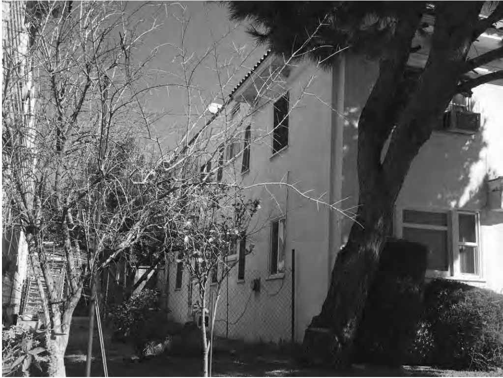
Figure 14: 4637-4643 Maubert Avenue, west elevation, looking northeast (GPA Consulting, 2019).
