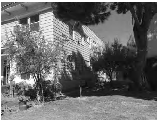
3. View of the east side of the subject property (building A), looking northwest.
