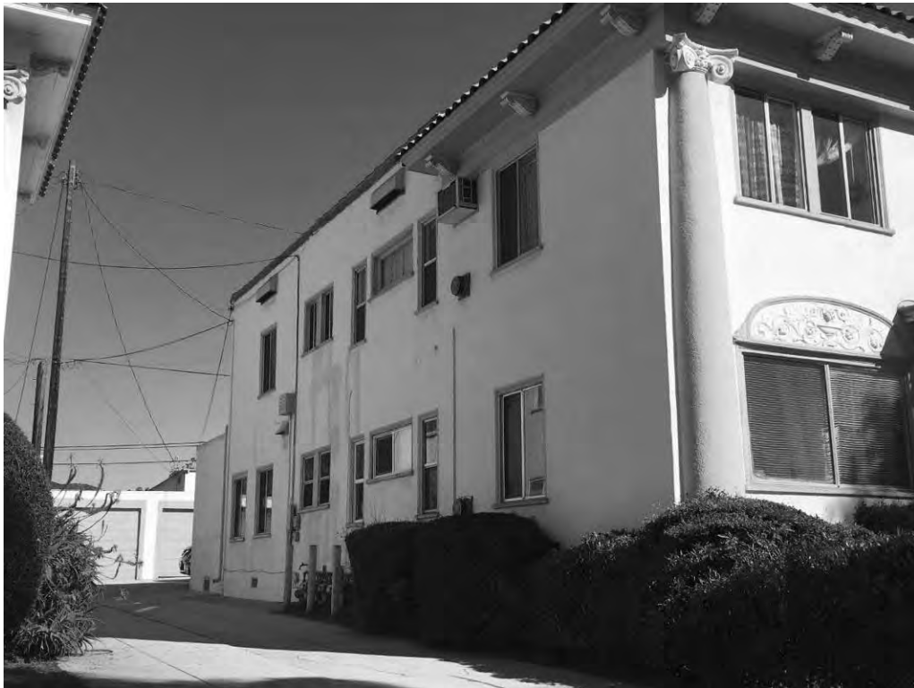
Figure 5: 4629-4635 Maubert Avenue, west elevation, looking northeast (GPA Consulting, 2019).
