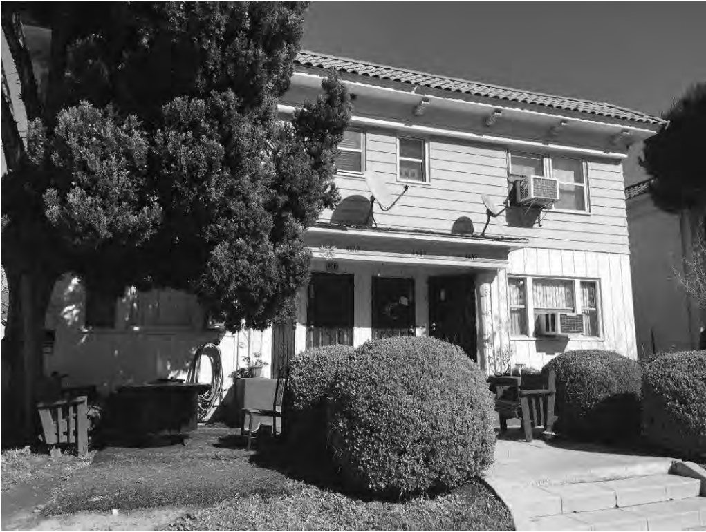
Figure 19: South elevation, looking northeast (GPA Consulting, 2019).
