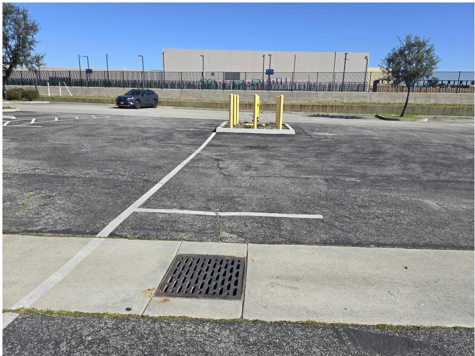
STORM DRAIN AND V-GUTTER
