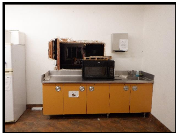
Looking at damage wall in kitchen.
