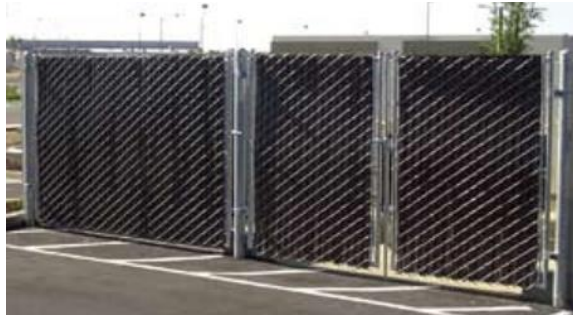
Image 1 – Chain-link fence with vinyl privacy slats
