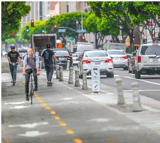
*Figure 12. Main & Spring Street Forward protected two-way bike lanes*
