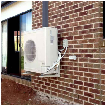
CONDENSING UNIT ON STAIR SHAFT WALL
